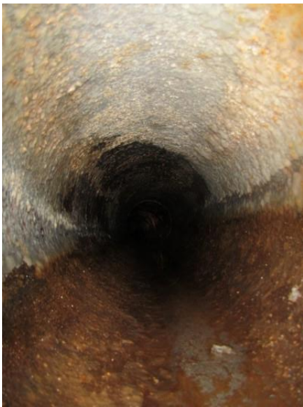
Photo C-13. Interior of Lakeline looking downstream
