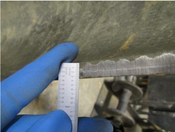
Figure 6.3-2 Graphitization on Interior Surface of Manhole 4 Sample
