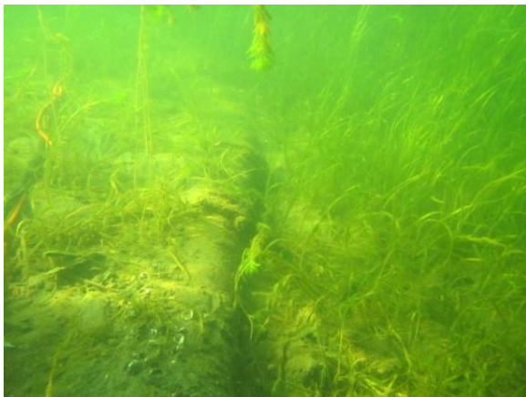
Photo C-54. Offshore side of mainline exposed
