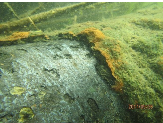
Figure 6.1-3 Surface of Mainline after Scaling and Corrosion Removed
