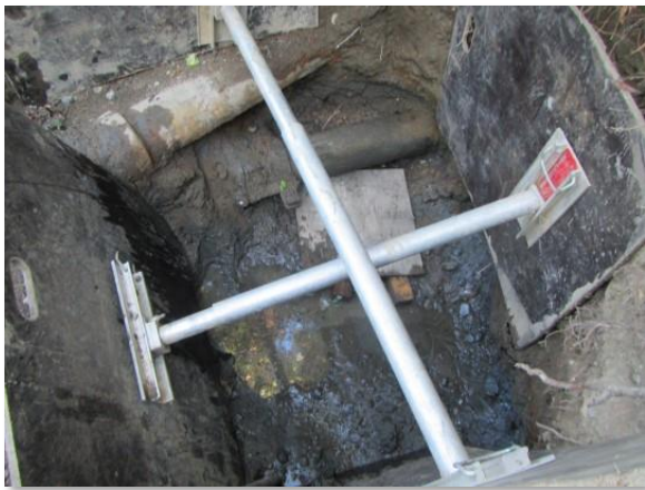
Photo C-1. Excavation pit; Lakeline below water main
