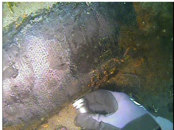
Photo 2-6. Typical pipe surface
