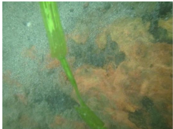
Photo C-36. Corrosion scale/tuberculation on individual pipe segments
