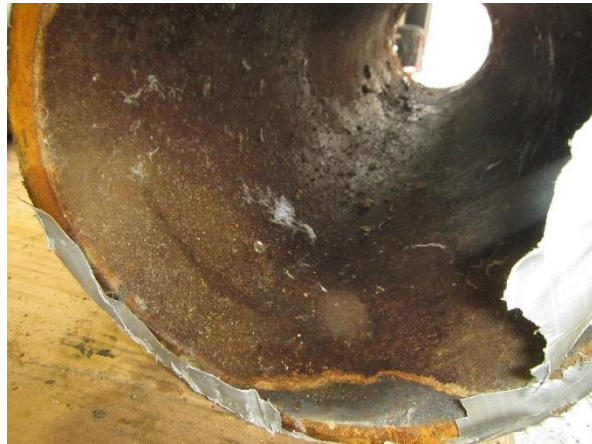
Figure 6.3-4 Cement Mortar Lining on Interior of Manhole 5 Sample
