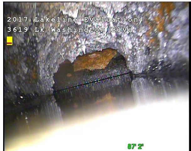
Photo 2-13. Wye or tee fitting connection to mainline at 3619 Lake Washington Blvd. North
