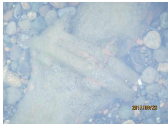
Photo C-42. Mechanical joint (first from shore)
