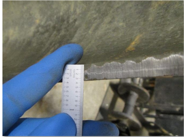
Photo 3-2. Graphitization on interior surface of Manhole 4 sample.
