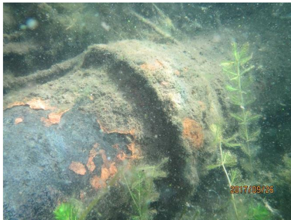
Photo 2-7. Typical bell and spigot joints between pipe segments
