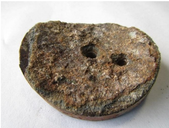
Figure 6.3-7 Deteriorated Cement Mortar Lining on Lateral Coupon
