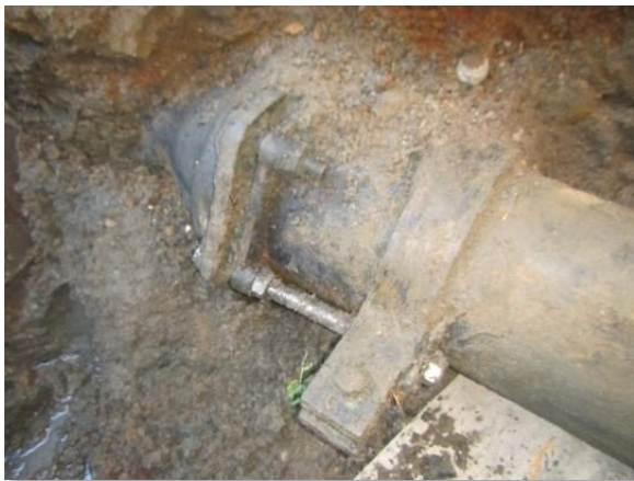
Photo C-7. 4"x8" reducer with mechanical joint
