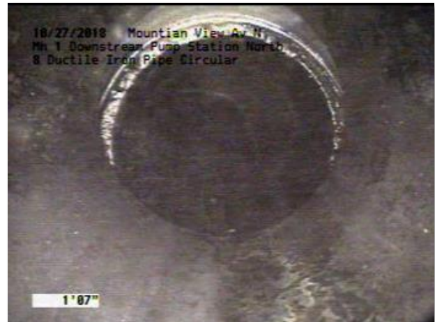
Photo 3-18. Typical offset joint.
