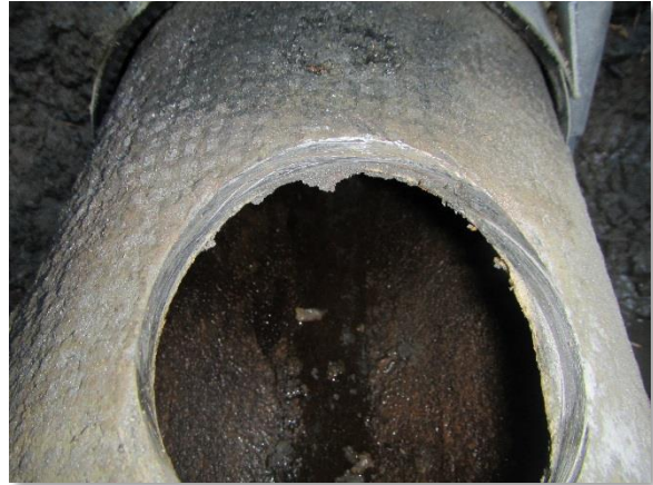
Photo 2-17. Pipe coupon hole
