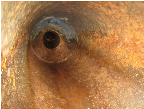
Photo C-11. Interior of Lakeline looking towards reducer
