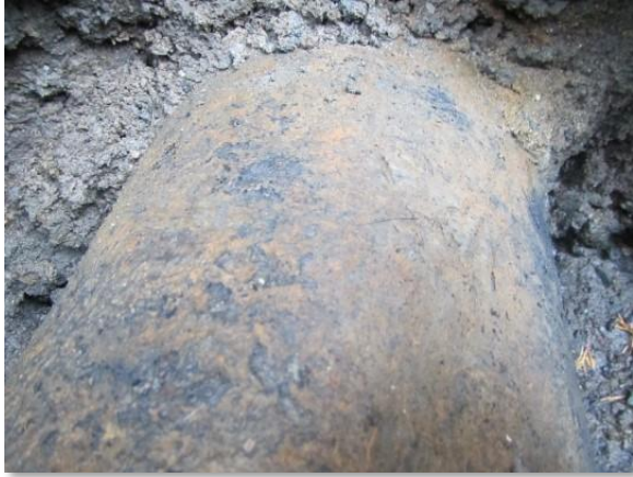
Photo C-3. Close up of top of Lakeline
