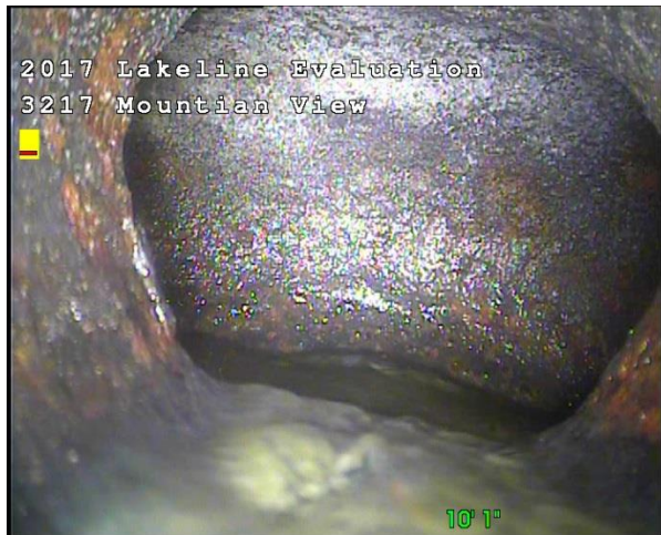
Photo 2-12. Wye or tee fitting connection to mainline at 3217 Mountain View Ave. North
