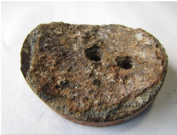
Photo 3-7. Deteriorated cement mortar lining on lateral coupon.
