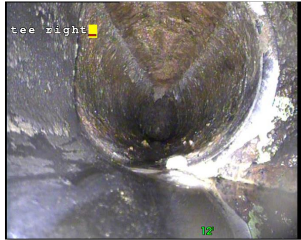
Photo 2-23. Apparent air pocket in lateral
