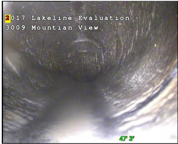
Photo 2-22. Typical lateral interior
